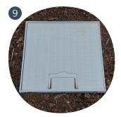
Position a proper size cover or grid over the catch basin and proceed with filling the lateral with terrain
