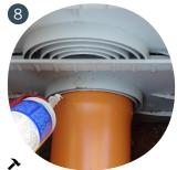
Seal the inlet/outlet tubes connection with silicone glue
