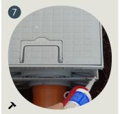
Seal the connection of the two catch basins with silicone glue
